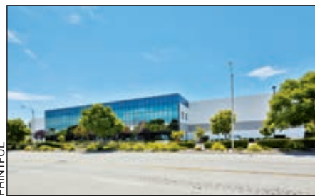
A 93,000-square-foot Valencia, Calif., facility (shown above) will open this fall to house on-demand-printing and drop-shipping-fulfillment business Printful.
