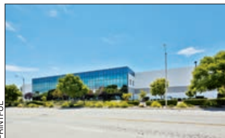
A 93,000-square-foot Valencia, Calif., facility (shown above) will open this fall to house on-demand-printing and drop-shipping-fulfillment business Printful.
